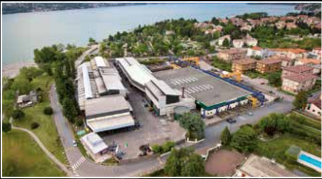
OFFICINE NICOLA GALPERTI E FIGLIO S.P.A. - FORGING PLANT I - ITALY
