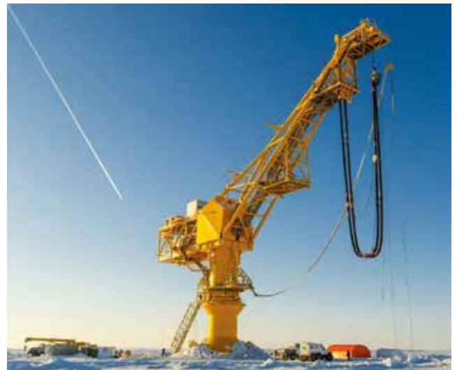
Arctic loading towers
